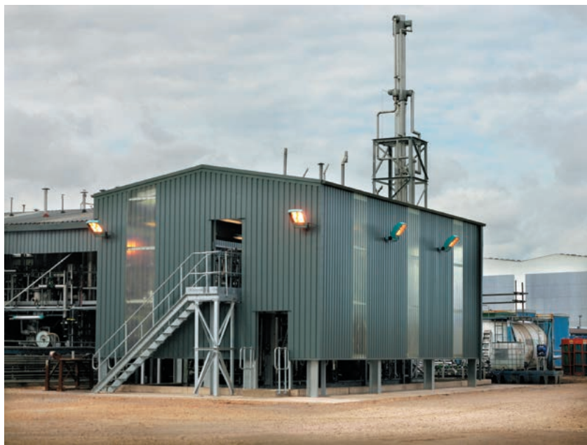
D1 Oils' new 10,000-tonne D120 Mark II, is a stand-alone skid-mounted continuous biodiesel refinery that can easily be shipped around the world by road, rail and sea. Photo courtesy D1 Oils plc.
