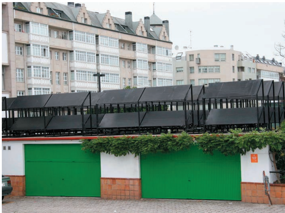
A Solar PST thermodynamic solar panel installation in Galicia, Spain. Photo courtesy Solar PST.
